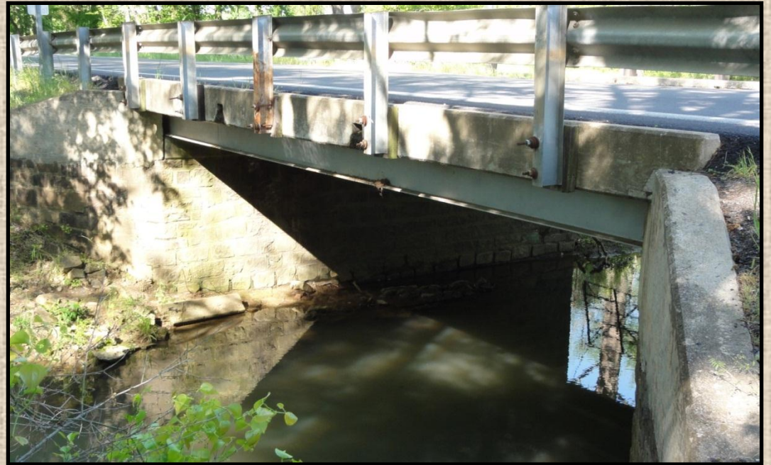
Evansville Creek Bridge
